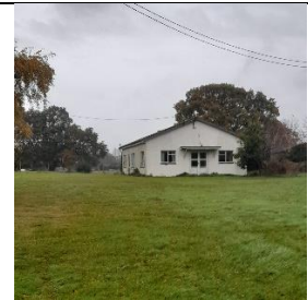
Asset 1 – Village Hall
